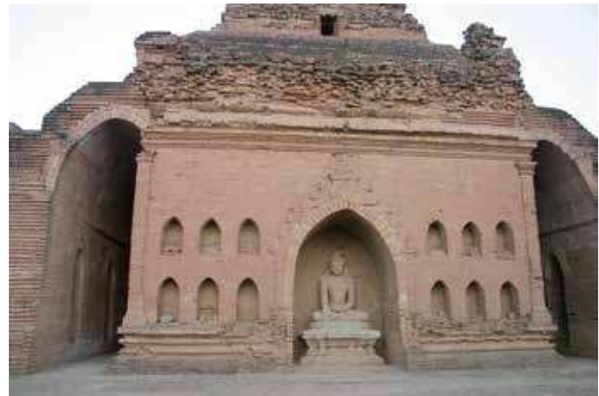
FIG. 35. The temple’s collapsed entrance hall has exposed the brick vaulting system. Pathadagu Temple, Pagan
